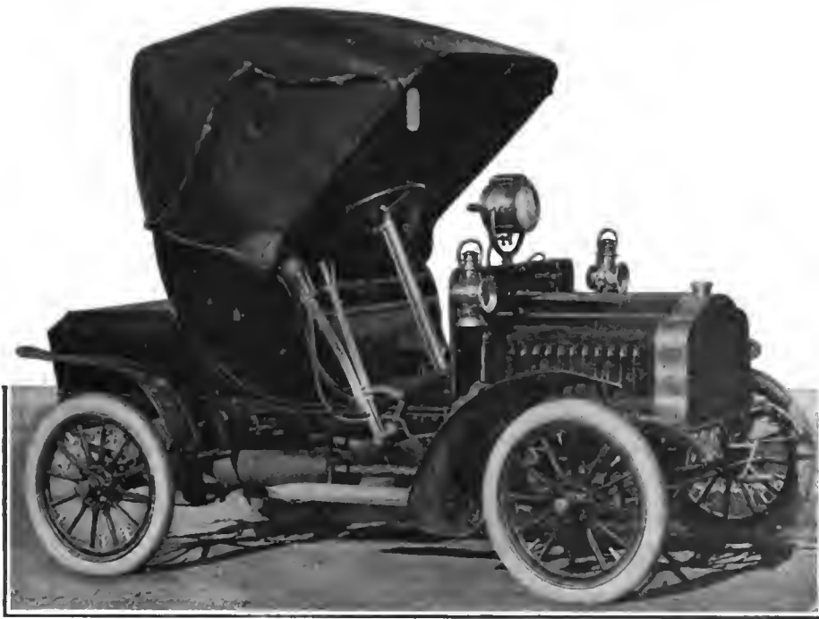
"DOCTOR COMPOUND" 15-HORSEPOWER CAR WITH STANHOPE TOP FOR PHYSICIAN'S USE.
